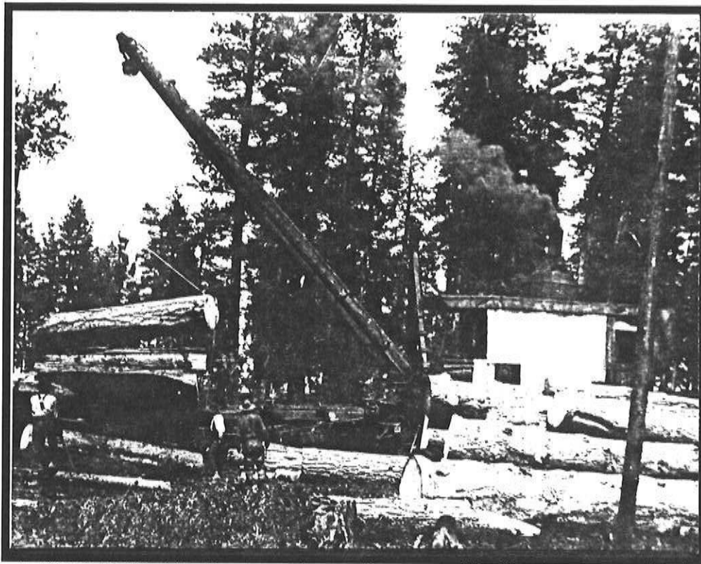
A "Steam Donkey" loading logs. A versatile means of loading logs on a railroad car. The steam donkey could be easily moved from one landing to the next. Mason Butte in 1921. (Photo: Winchester State Park)
