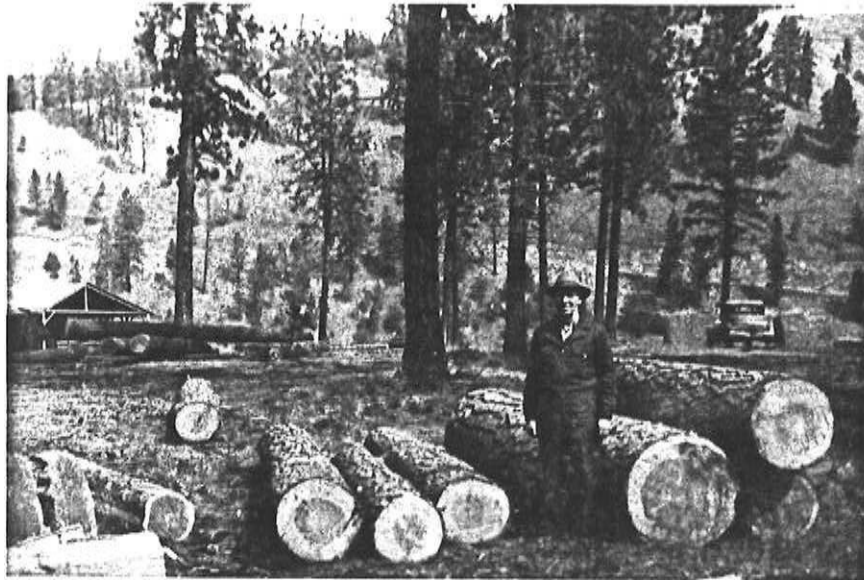
Ranger Norton with logs from the Gilbert Grade Unit during another war-time timber sale, March 1944. (Photo: National Archives, Seattle Branch)
