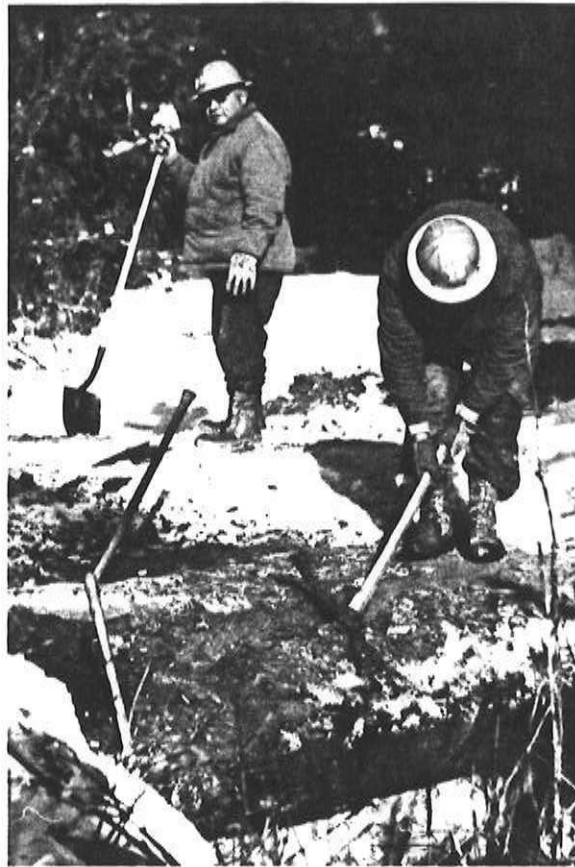
APW road crew (Herman Reuben, Jim Andrews, Aaron Ramsey) replacing a log culvert. Tramway Reserve, 1965. (Photo: BIA, Northern Idaho Agency)
