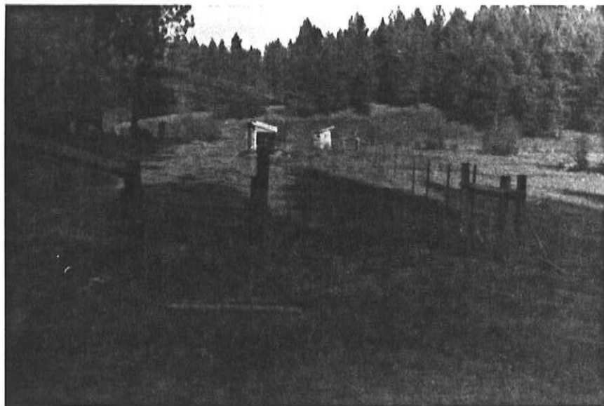
Fence and gate around a campground. Installed as an APW project. Mud Springs Reserve, 1965. (Photo: BIA, Northern Idaho Agency)
