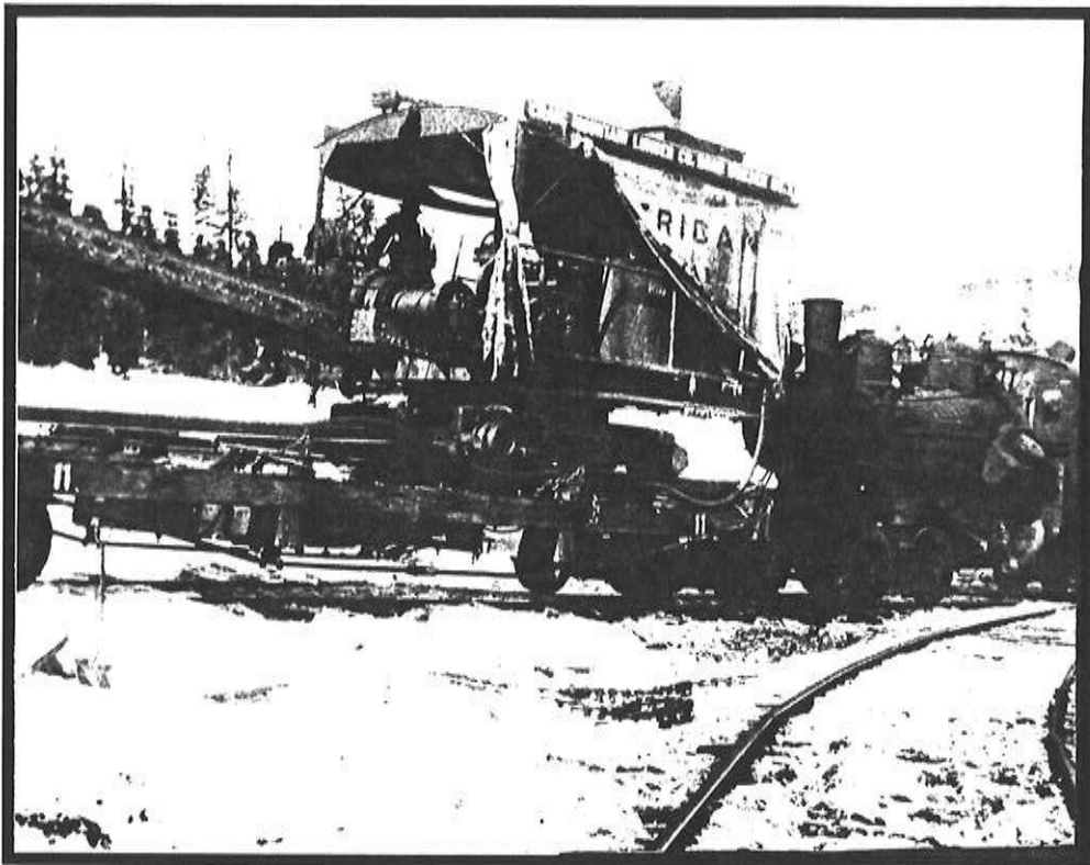
A common form of transportation in the 1920s was railroad. Railroad tracks were laid by this Craig Mountain Lumber Company Road Builder No. 1 into every possible timbered parcel. This railroad was narrow gauge using "work" engines such as the one pictured. Mason Butte, 1921. (Source: T. Roberts, Nez Perce Tribal Forestry Office. Photo: Winchester State Park)
